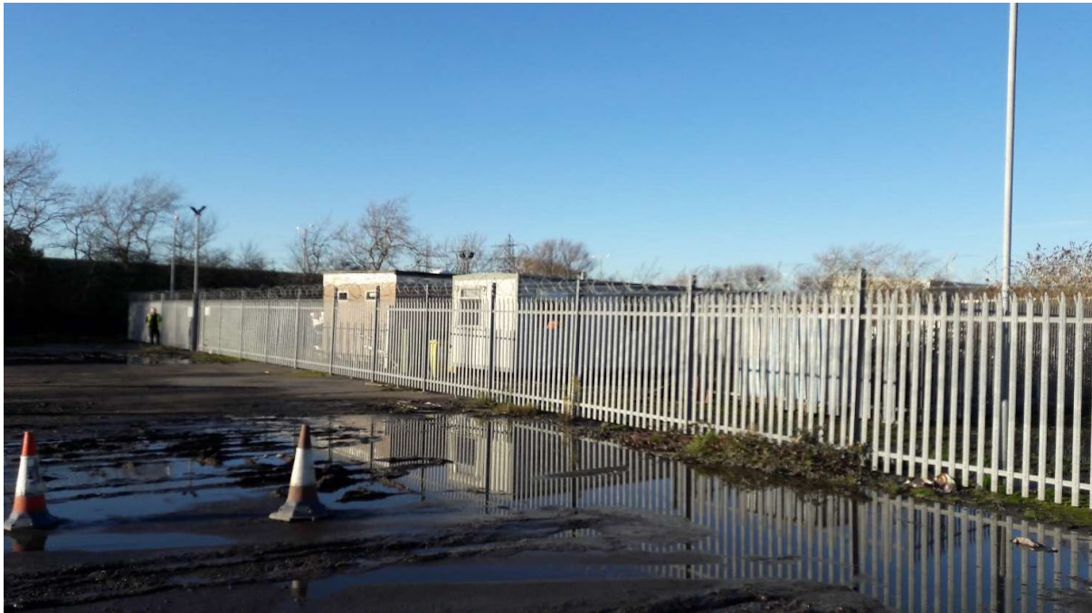
Figure 4: View from the temporary construction area into the proposed site showing temporary buildings
